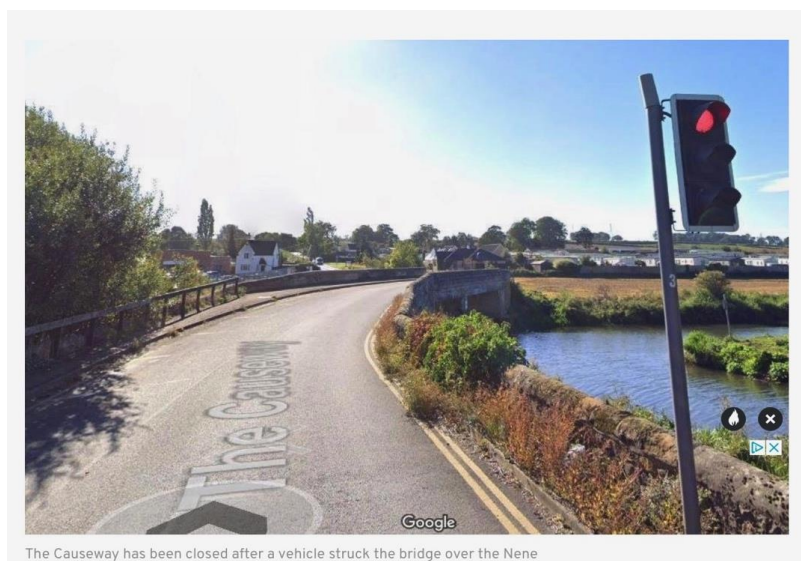
The Causeway has been closed after a vehicle struck the bridge over the Nene
